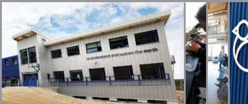
Leading-edge design at the remote Churchill Northern Studies Centre lowers operational costs, and increases utility reliability and independence
