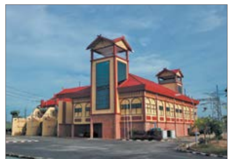
Thailand-Malaysia HVDC Converter Station (Thailand)
