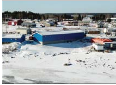
Pauingassi First Nation Water Treatment Plant
